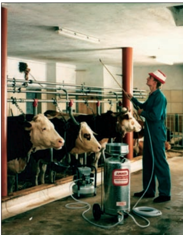
Figure 5: Example of whitewashing of a stable with milk of lime. Milk of lime may also be applied by brush or other suitable technique (Austria).
